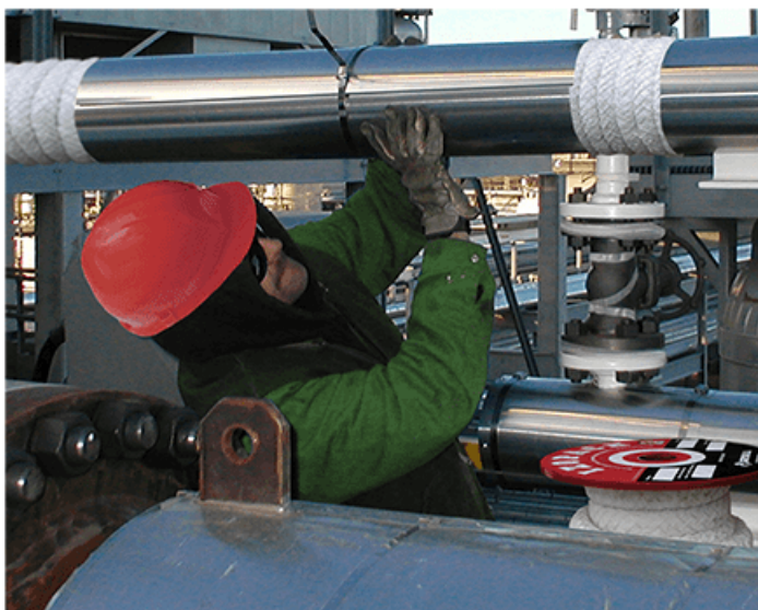
1 - cord IZOPACK; 2 - wire mount; 3 - thermal insulation fabric; 4 - yarns; 5 - mounting of jacket by wire or clamps; 6 - outer jacket
